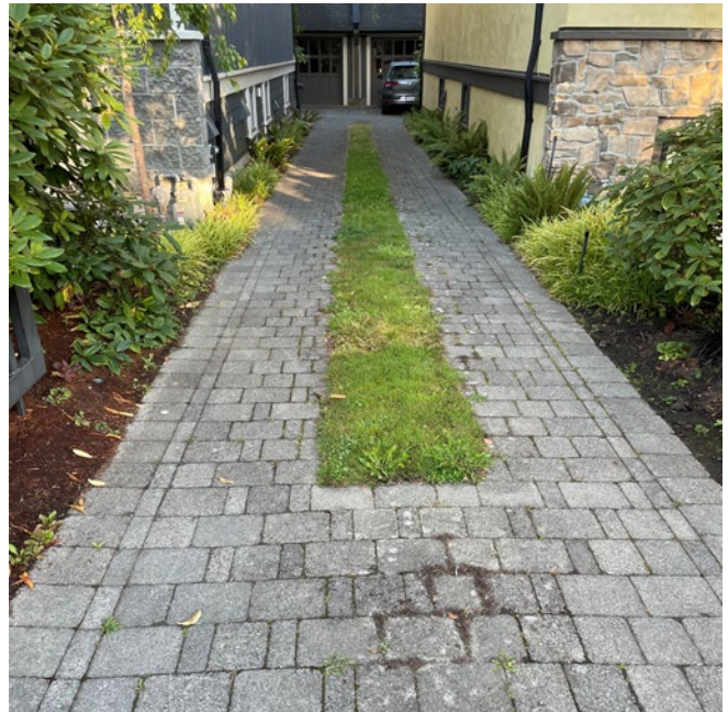
Figure 13. An ingenious approach to permeable paving, where car-related contaminants are captured in the vegetation and soil before entering nearby storm drains. Photo by Kyla Sheehan.
