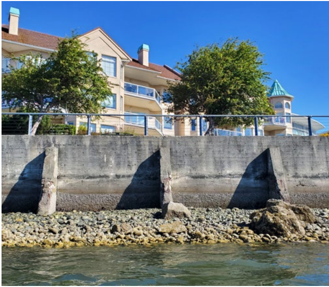
Figure 6. Seawalls are fixed structures on our coasts, preventing habitat from adjusting with changing conditions. Photo by Maria Catanzaro.
