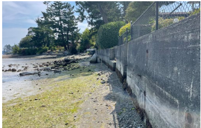
Figure 9. Armoured shorelines tend to cut off the intertidal habitat, reducing diversity of the shore.
