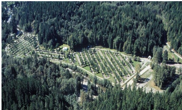
Weaver Creek Spawning Channel, aerial view looking northwest.
